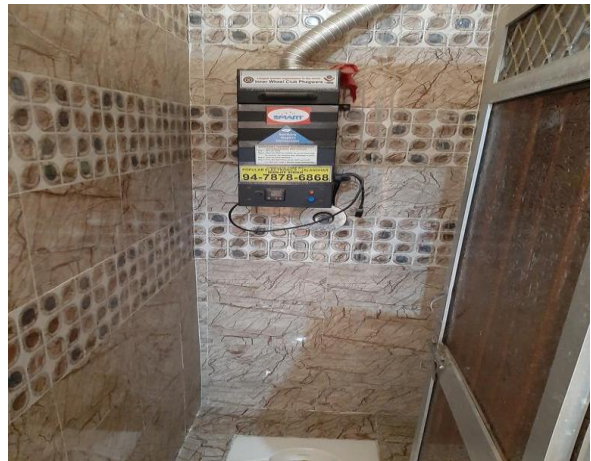
Waste Recycling System (7.1.3)
