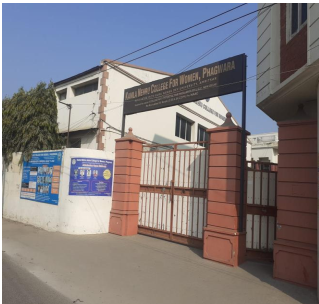
Net Wall Compound (Safety & Security (7.1.1)
